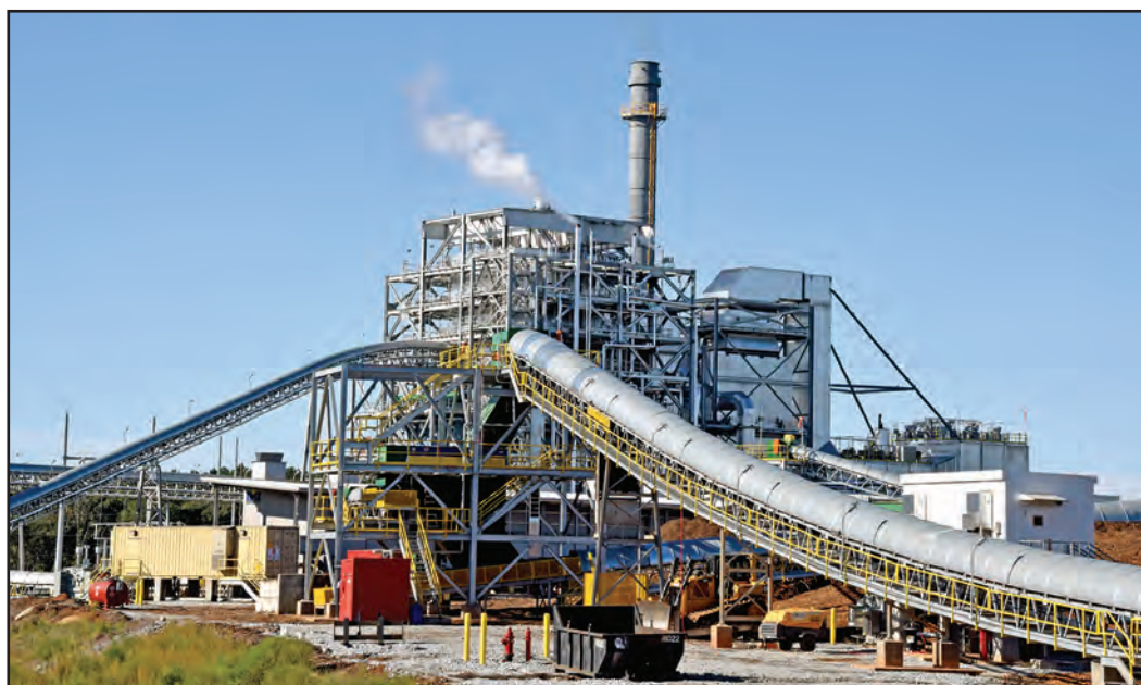
The Franklin County GRP plant (above) near Carnesville is part of a suit that alleges the owners of it and other plants misrepresented financial information to get help with foreign investment.
